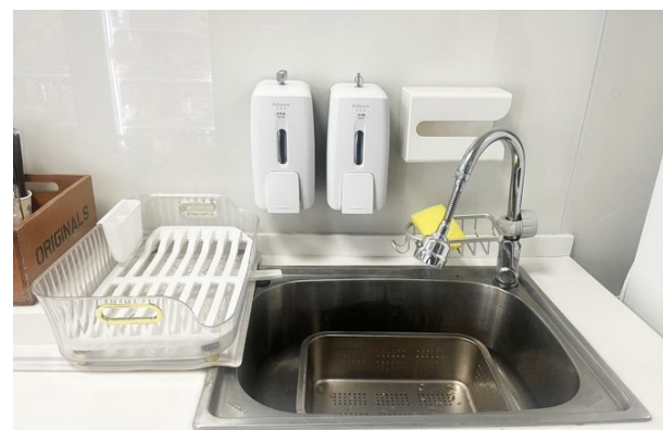
Installed Water Savers on Faucets
